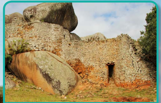
In some sections of the ruins, giant boulders were incorporated into the strong brick walls.
