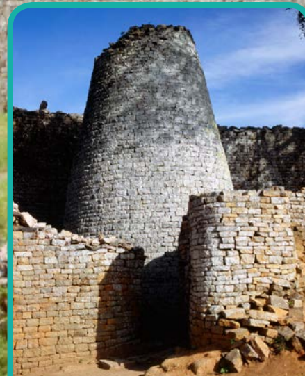
The builders of Great Zimbabwe erected very high brick walls without the use of mortar by layering the bricks on a slightly inward slope.
